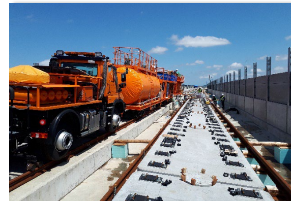
Hokuriku Shinkansen Fukui track construction
