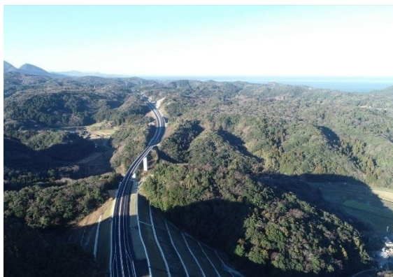
FY2022 Shizuma Nima Road pavement construction work in Isotake district (Chugoku Regional Development Bureau, MLIT)
