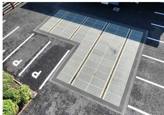
OKS Company's Wattway, pavement with a solar power generation function
