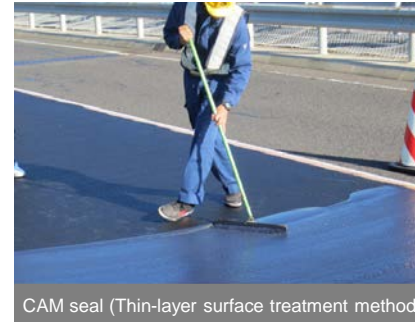
CAM seal (Thin-layer surface treatment method)
